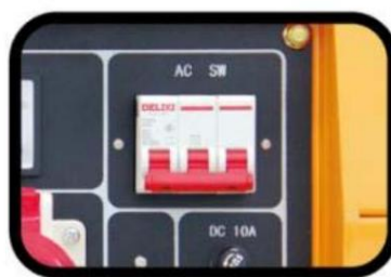
STEP 3. Turn the circuit breaker off.
